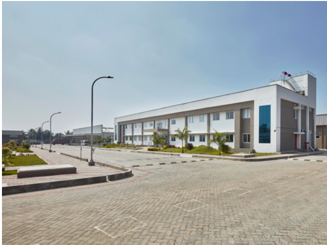
Manufacturing Facility at K R Pete, Mandya, Karnataka
